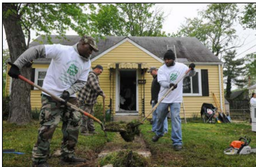
Volunteers from the 113th Wing came together to make repairs to the home of Grace Williams, 75, as part of the Prince George's County's Christmas in April program in Forestville, MD, April 30. The program allowed for the members of the DCANG to give back to their community and help those in need.
