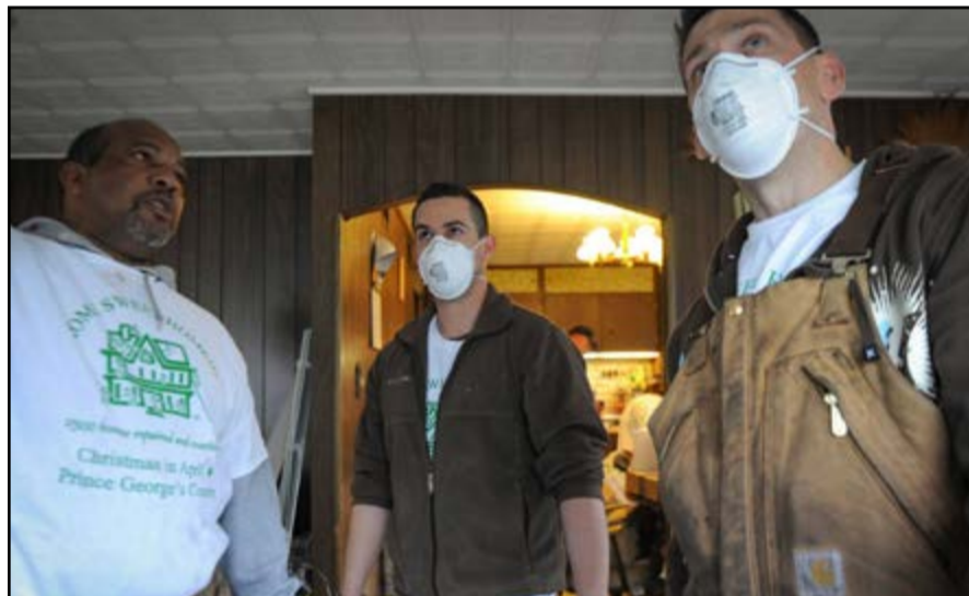
113th Wing Civil Engineering Squadron members Larry Countiss, Capt. Matt Duller and Senior Master Sgt. Sterlin Wilson assess the repair needs of an interior wall Saturday, April 30, 2016 during a Christmas In April renovation project in Forestville, Maryland.
