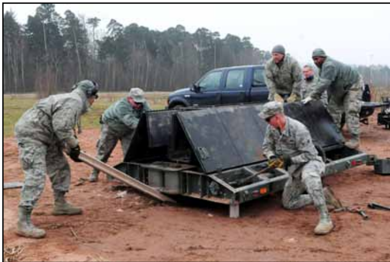
Power production technicians prepare a mobile runway edge sheave for removal during training in Silver Flag 2016 at Ramstein Air Base, March 11. The Mobile Aircraft Arresting System is used in contingency environments allowing aircraft to safely land in the event of an emergency or where conditions are not present for conventional landings.
